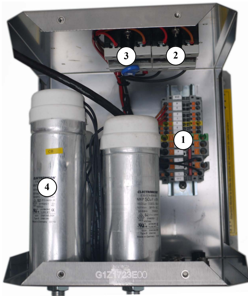
Fig. 5.14.2-1: AC-Control box single phase - example
