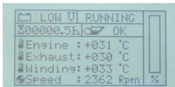
Fig. 18.1.1-1: Warning: „Battery power too low“
