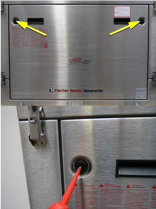
Fig. 3.5-1: Sound insulation capsule, side part
